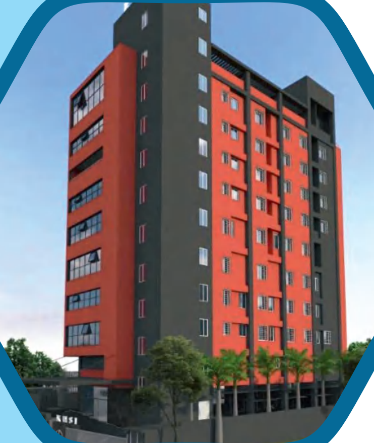
UROKUL, Baner, Mumbai -Pune Highway, Next to Bitwise, Pune
